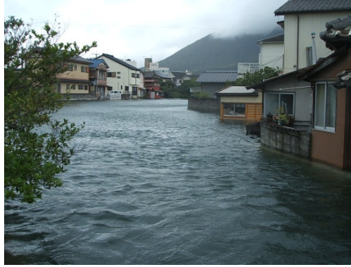
Fig. 2 Effects of TY Sanba (1216). Storm surge in Nagasaki Prefecture(photo: Shimabara City).
